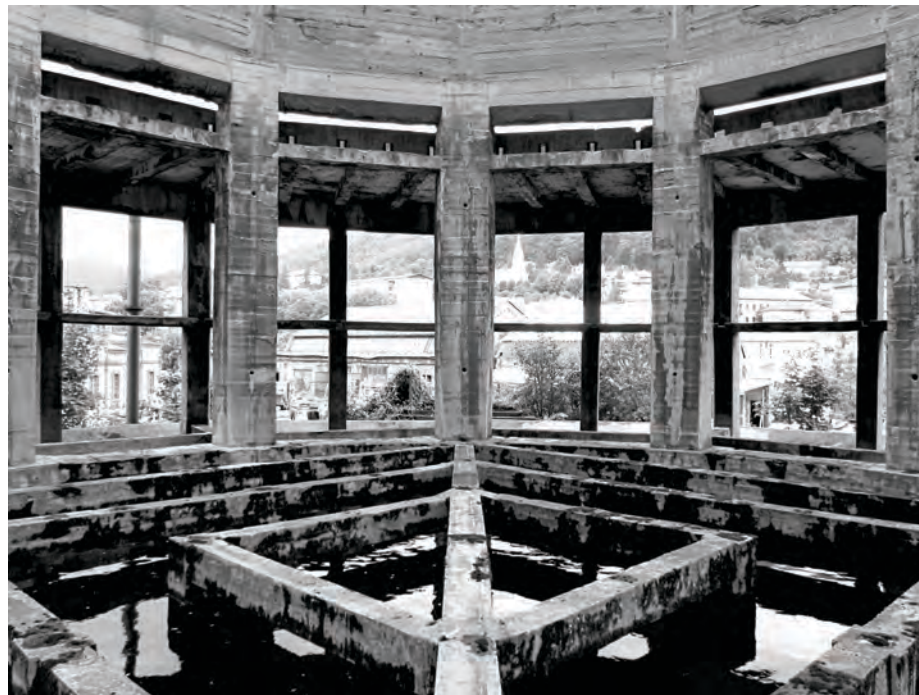
Dreapta / Right: Turnul de apă al centralei electrice | Water tower from the power station
